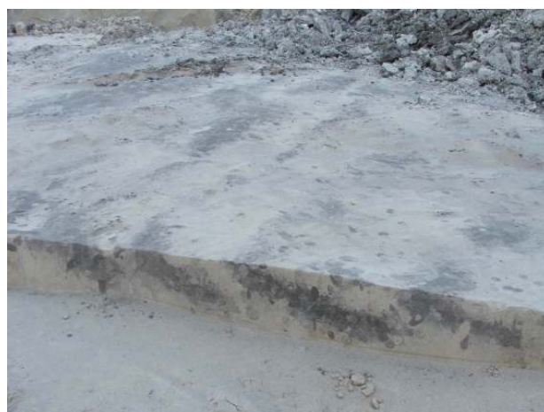
Fig. 9 Plough marks stretching from north to south (foto: Szabolcs Rosta)
