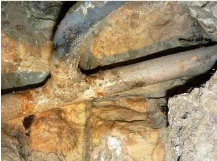
*Photo 2. Exploration of worn corroded pipes in concrete-stone foundation*
